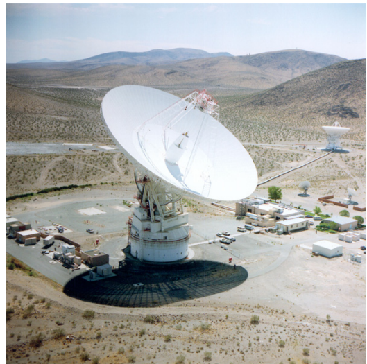
Fig. 1: The 70m antenna at the Deep Space Network Goldstone complex in the California Mojave desert. At the right can be seen one of the 34m antennas.
